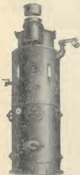
CRADLEY PATENT VERTICAL MULTI- TUBULAR BOILER
