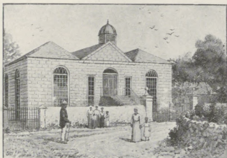
HAMPDEN CHURCH (FRONT VIEW), SHOWING ENTRANCE TO GALLERY.
