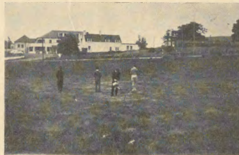
Spreading weed killer on the project site
