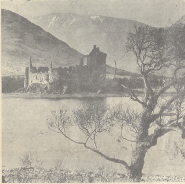
Kilchurn Castle, Loch Awe, from the south, with the remnants of the winter's first fall of snow on the hills.
