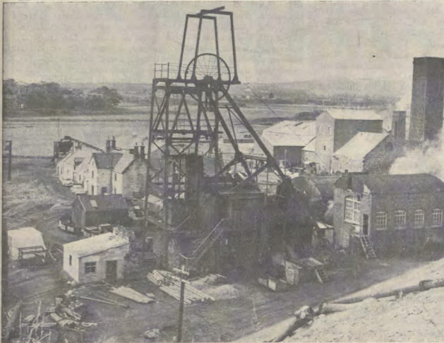
The now silent Brora Coal Mine by mid-winter will be producing more coal than ever before. The faith and perseverance of the miner-owners pays off.
