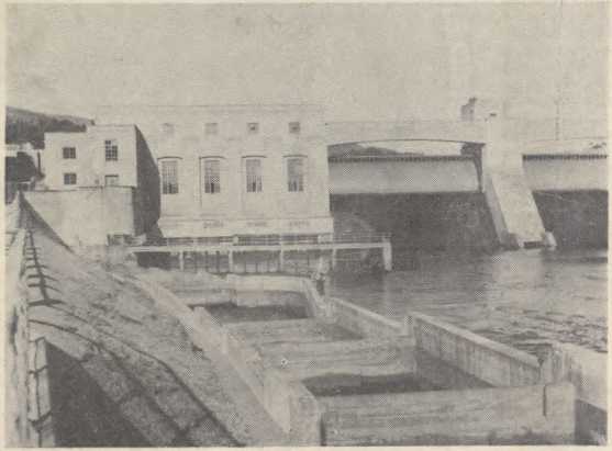
Fish Ladder, Pitlochry — An example of a Hydro Board construction designed to allow salmon to reach the upper stretches of the river to spawn. The dam is 900 ft. long and has 35 pools.
