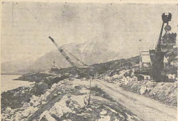
Work in progress on the Invergarry/Kyle road. This section has now been completed.
