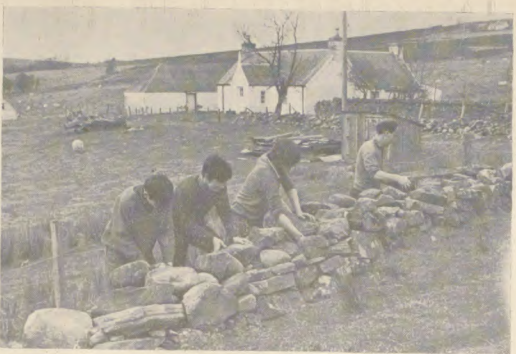
Rebuilding a dry-stone dyke
