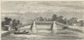
Bridge near Shanghai.
