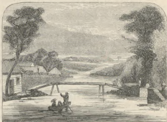
Bridge near Tsing-poo.
