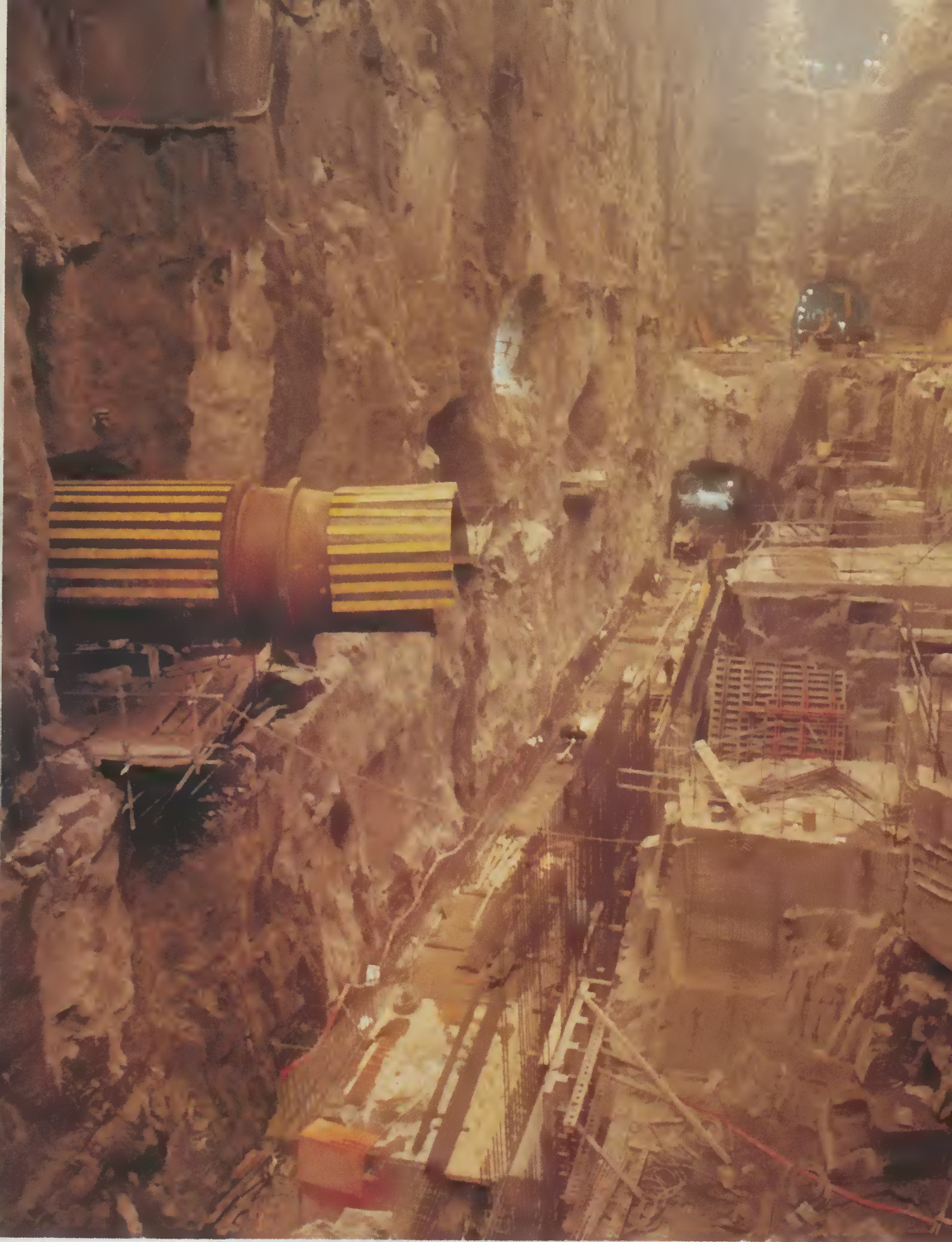
One of the world's largest man-made caverns which will house the main plant of the Dinorwic pumped-storage power station in North Wales; three million tons of slate have been hewn out of a mountain but after landscaping all that will be seen of the project is a door in the mountainside. When completed, Dinorwic will be able to contribute 1,320 MW to the national grid within ten seconds of demand.
