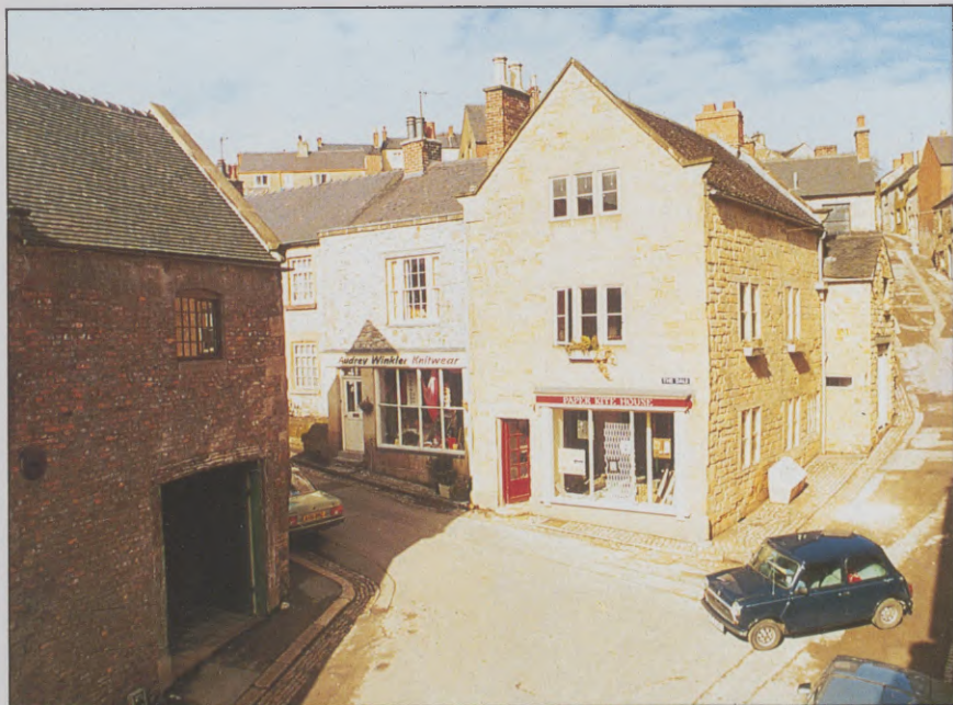
Restoration of Greenhill and The Dale, Wirksworth, Derbyshire.
