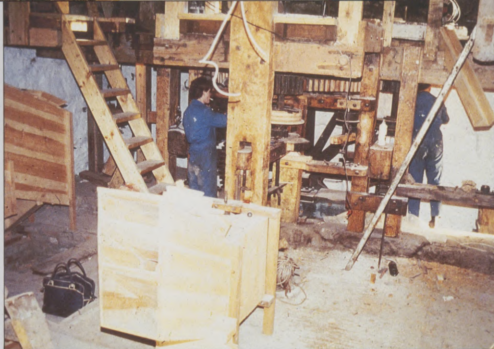
Annalong Cornmill restoration, County Down.
