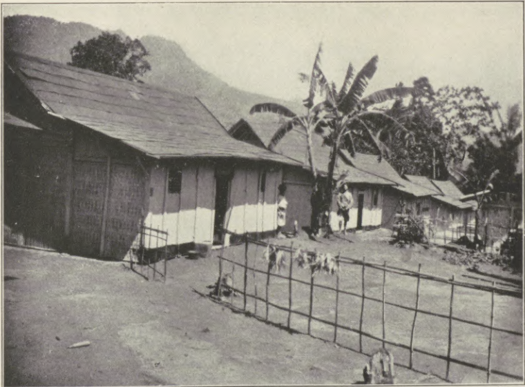
Figure 20. — The same complex after improvement.
