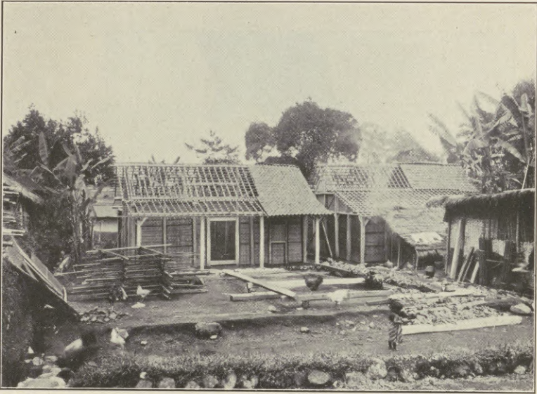
Figure 21. — Manner of joining architrave beams.
