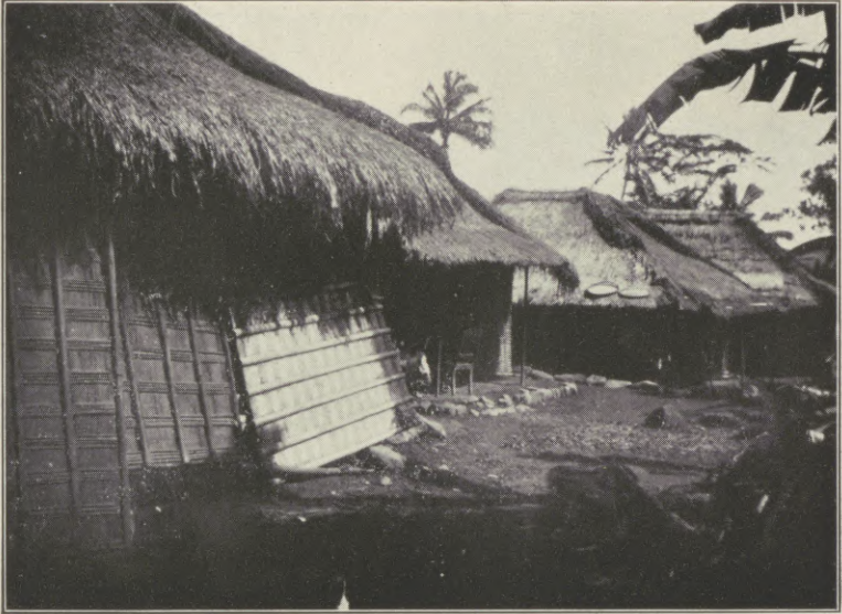
Figure 19. — A house complex prior to improvement.
