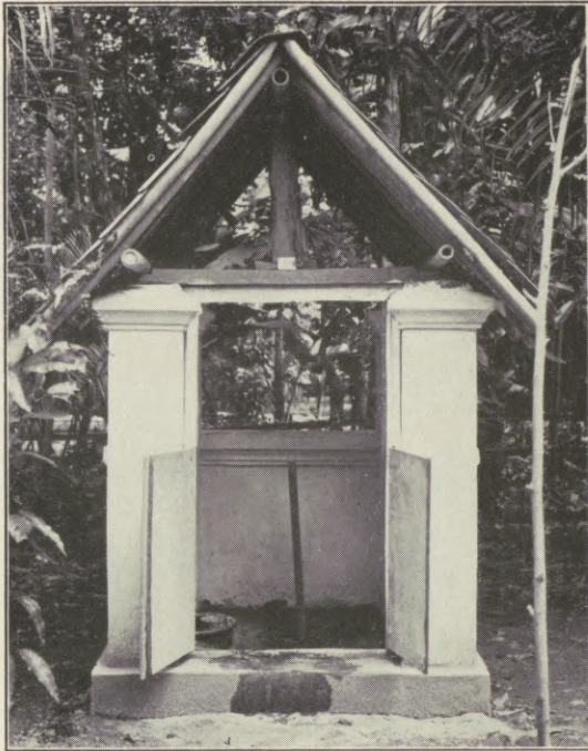
Figure 11. — Bored-hole latrine with cement floor and brick superstructure.
