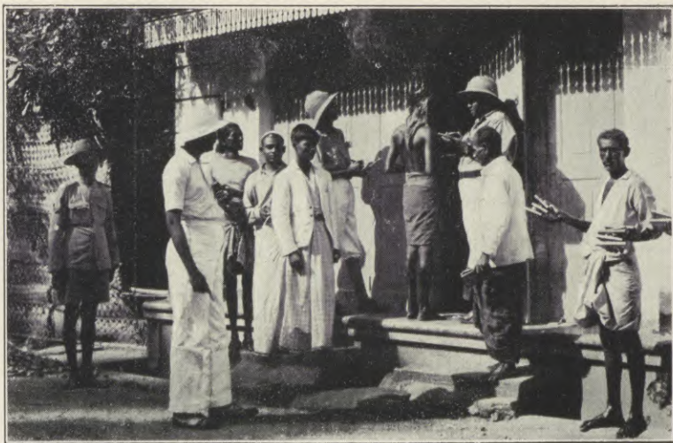
Figure 12. — Laying of rat-traps in buildings.
