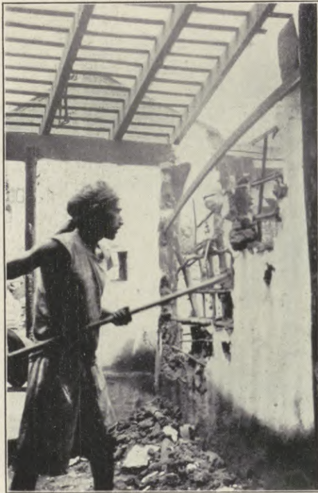
Figure 15. — Breaking-down of rat harbourages—wattle-and-daub walls.
