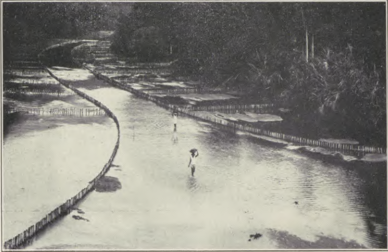
Figure 8. — Bamboo stake fences and channel cross dikes.
