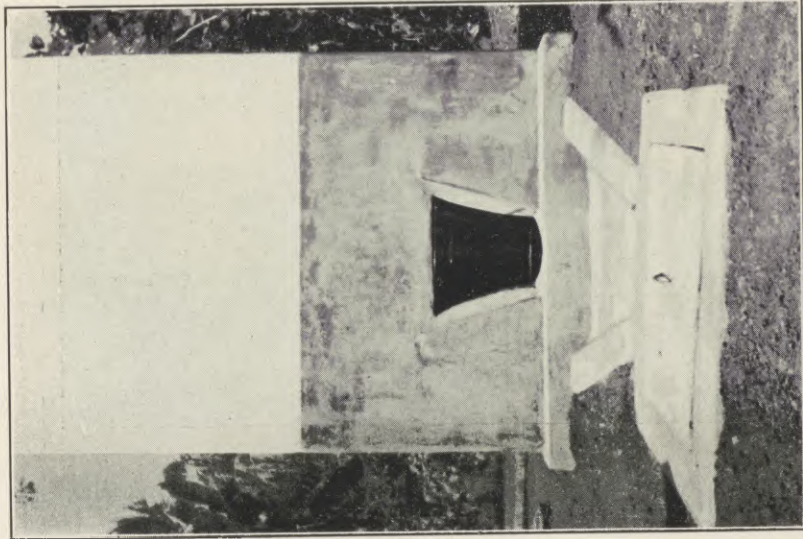
Figure 3. — Bucket latrine; bucket chamber conforming to shape and size of standard-size bucket, and sealed pit for disposal of wash-water.
