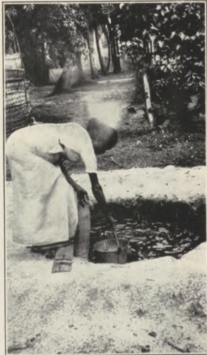
Figure 7. — Unbuilt dug well: anopheles breeding-place.
