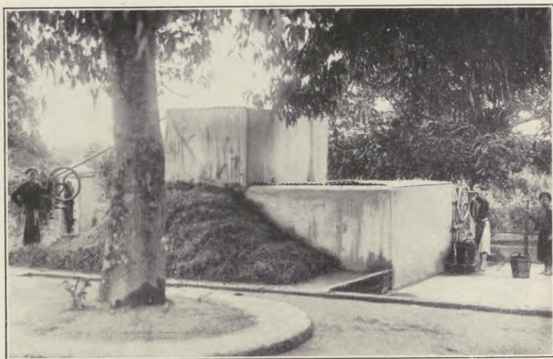
Figure 14. — Cement well and reservoir built by a village (province of Hadong, Tongking).
