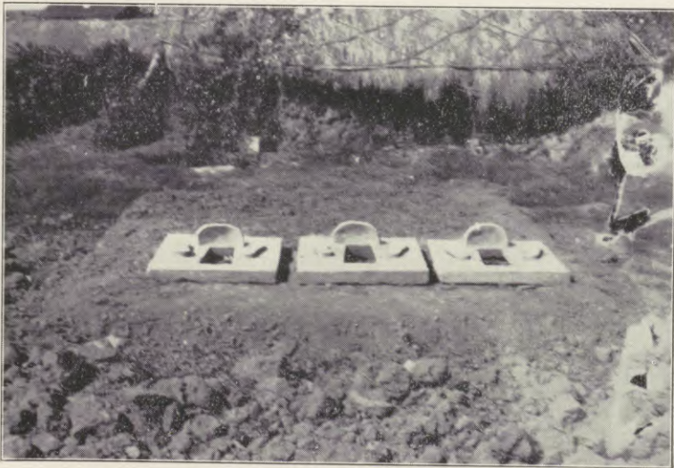
Figure 23. — Bored-hole latrine showing squatting-plates.
