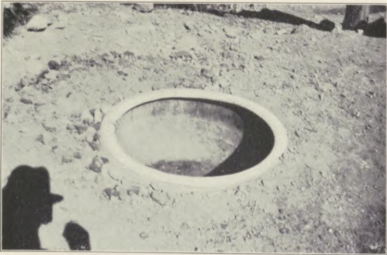
Figure 14. — Large earthenware jar for storing night-soil.
