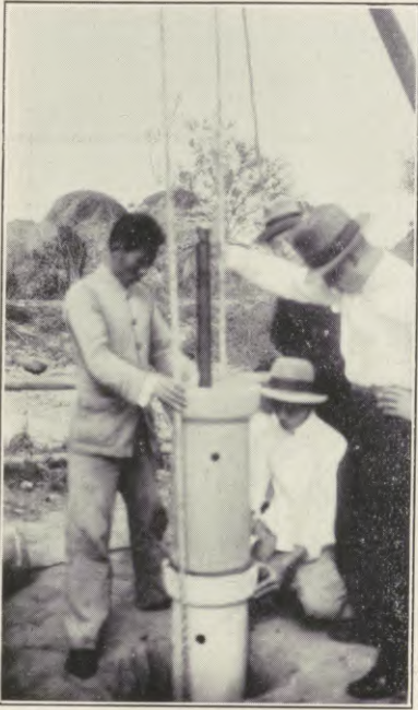
Figure 21. — A close-up view of the well construction.
