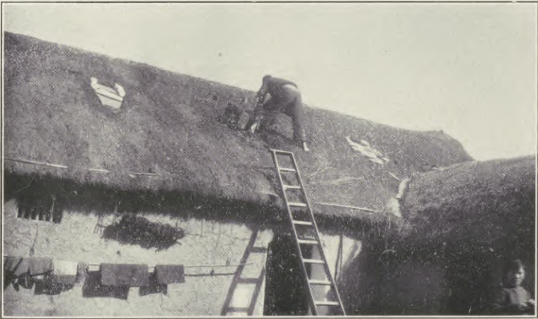
Figure 16. — Inserting skylights in a roof.
