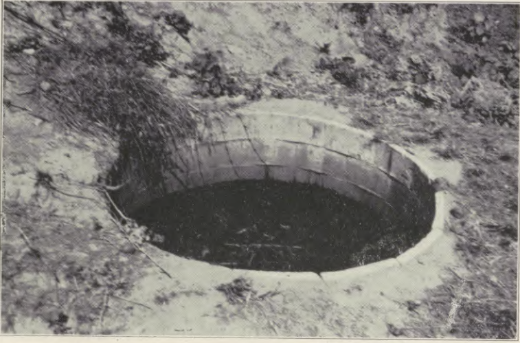
Figure 13. — Brick-paved pit for storing night-soil.
