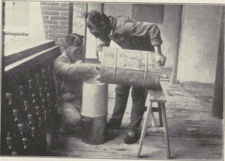
Figure 27. — Transferring cyanogas dust from a large to a small drum. Note the gas-masks.
