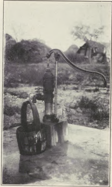
Figure 22. — A village hand-pump. Note the concrete apron surrounding the well.
