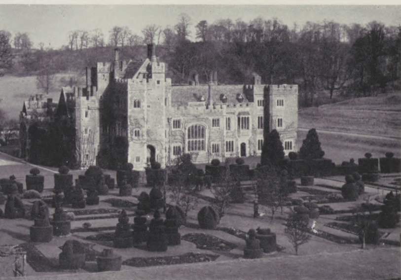
Compton Wynates. This early Tudor house in Warwickshire is about 200 years older than Chatsworth.
