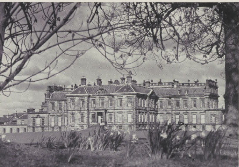
Hopetoun House. This mid-eighteenth-century Georgian mansion near Edinburgh has received a grant from the Historic Buildings Council (see p. 428).
