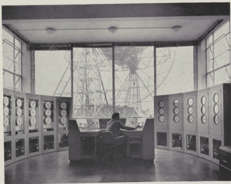
The control room and computers. The telescope will be floodlit by night.
