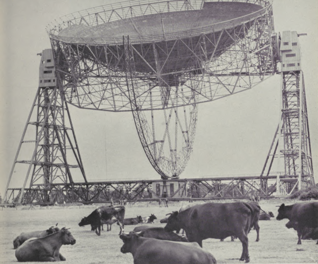
The world's largest steerable pencil-beam radio telescope at Jodrell Bank (see pp. 409 and 422). It has an estimated reach of 1,000 million light years; the reflector bowl, 250 feet across, rests on 180-foot towers which rotate on a track 352 feet in diameter.
