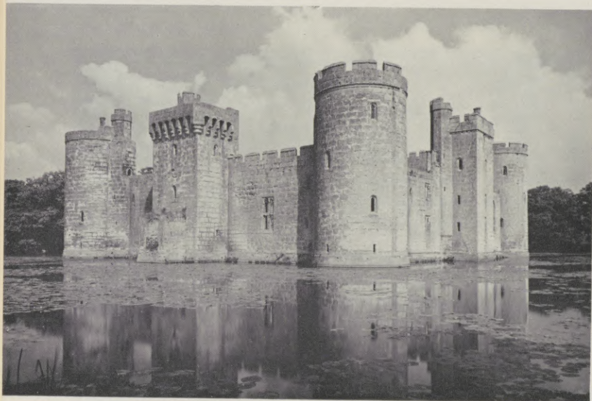
Bodiam Castle in Sussex, built about 1386, is one of several English castles owned by the National Trust (see p. 215).
