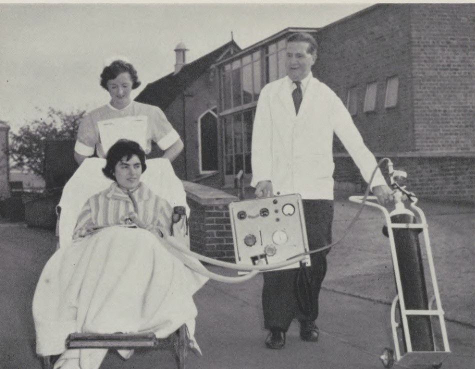
The Barnet Ventilator is a 56-lb. portable electronic lung developed in Britain for use in the treatment of respiratory conditions such as poliomyelitis.
