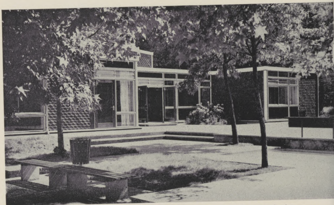
A primary school built under the CLASP prefabrication system developed by Nottinghamshire County Council.
