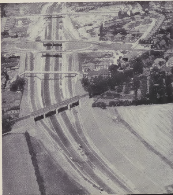
Doncaster-Sheffield Motorway at Warmsworth.
