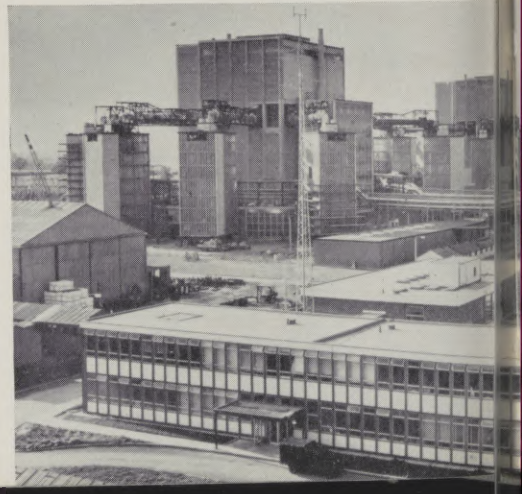
Berkeley Nuclear Power Station (started operation in 1962).
