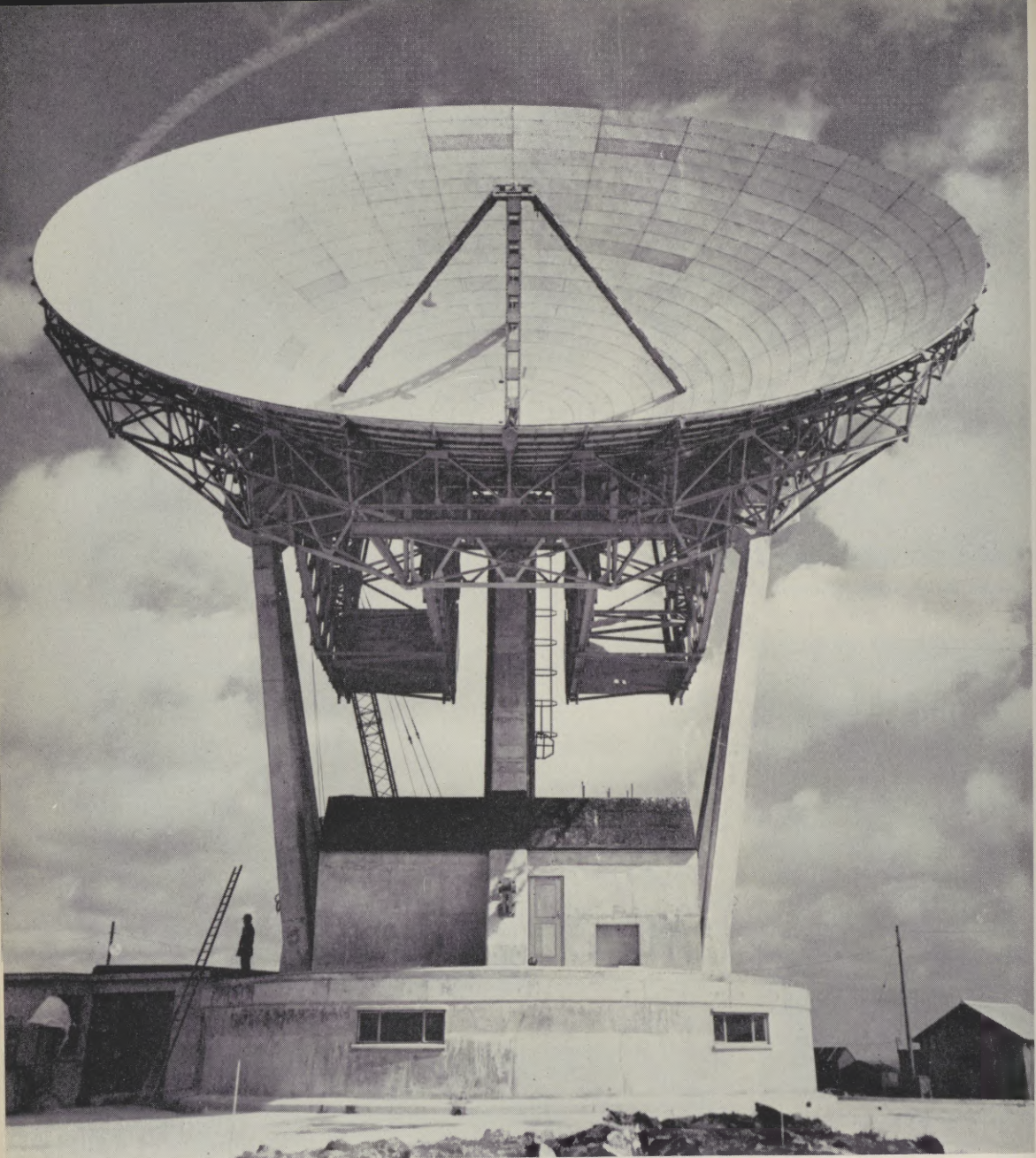
The Post Office satellite communications ground station at Goonhilly Downs, Cornwall (see p. 217), by means of which the first experimental live transatlantic television pictures were exchanged between Britain and the United States via the US satellite Telstar in July 1962. The steerable aerial has an aperture diameter of 85 feet.
