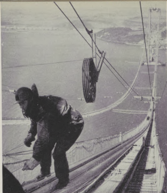
Forth Road Bridge under construction.
