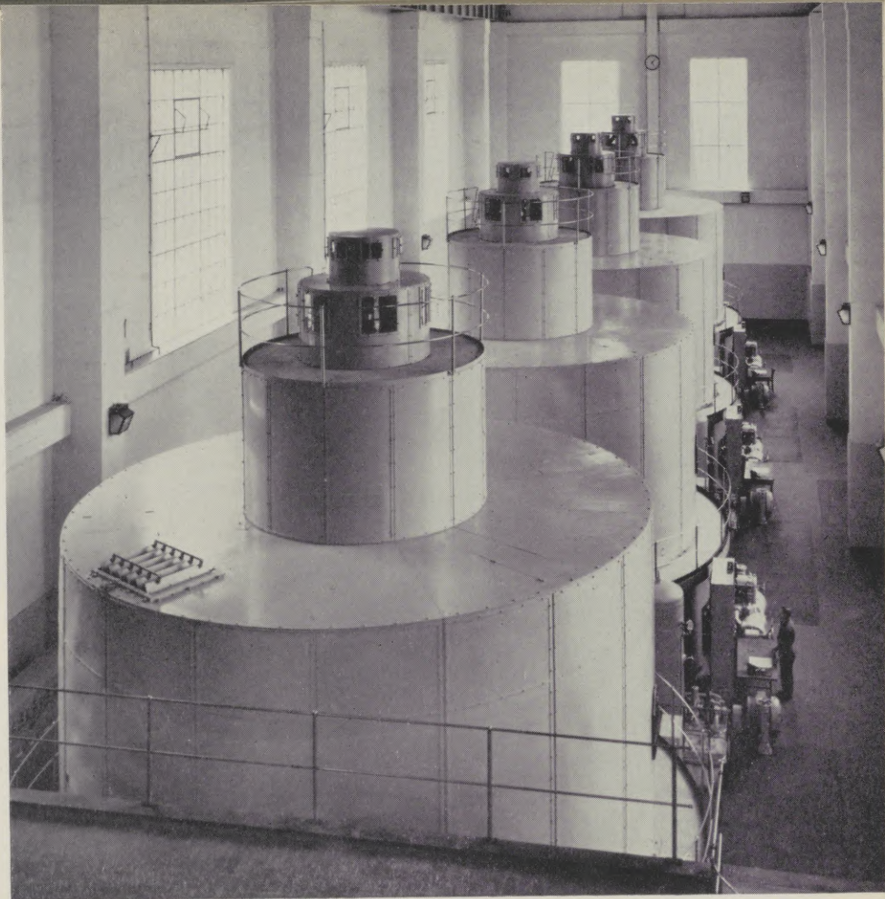
English Electric Company's 45,500 h.p. turbines at the Loch Sloy power station (North of Scotland Hydro-Electric Board).
