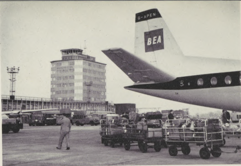
The new control tower at Ringway airport, Manchester.
