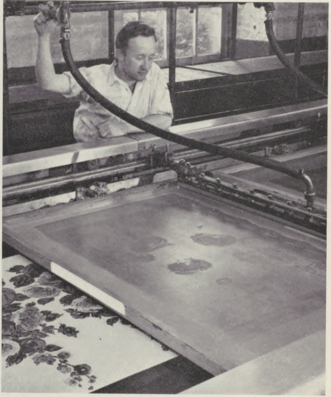
Automatic screen printing for cotton fabrics.
