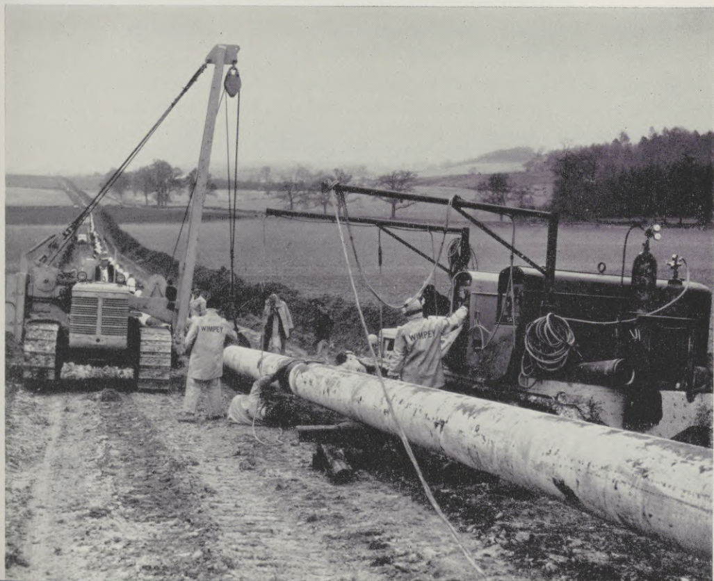
Laying a section of methane pipeline.
