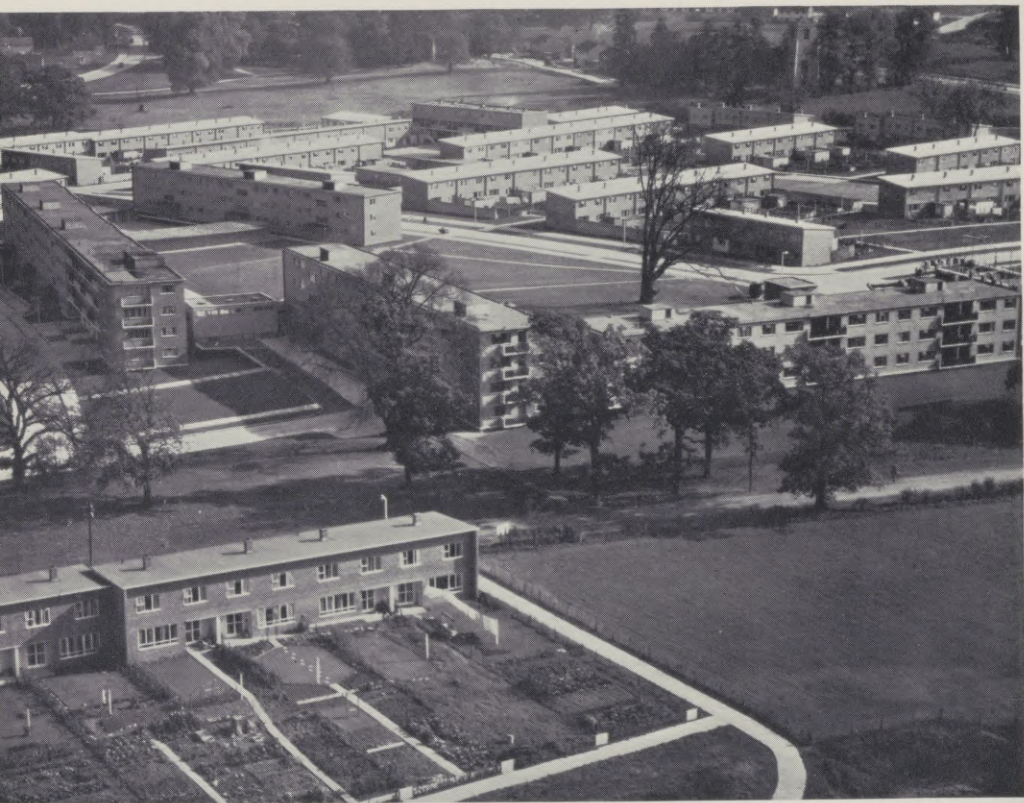
Houses and flats at Harlow, Essex, one of the eight New Towns near London (see p. 330).
