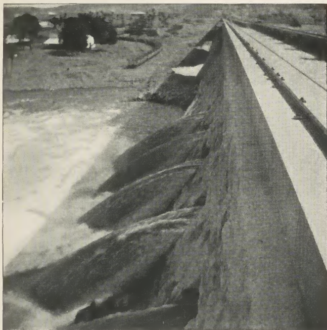
FIG. 5A.—Front of Assuan Dam, from above.
