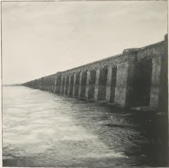
FIG. 2A.—Assiut Barrage, downstream side.
