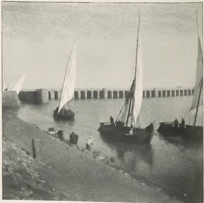
FIG. 2B.—Assiut Barrage, upstream side.
