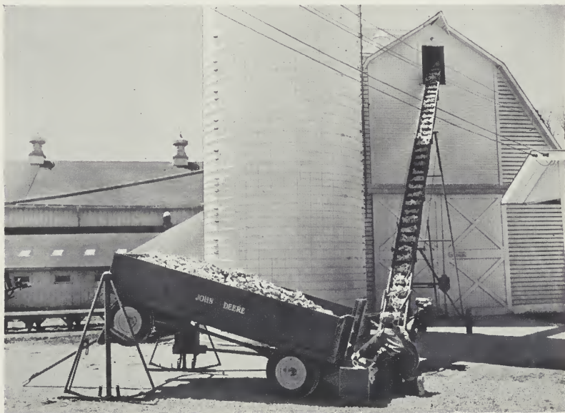
Plate 5 Chain and flight elevator
