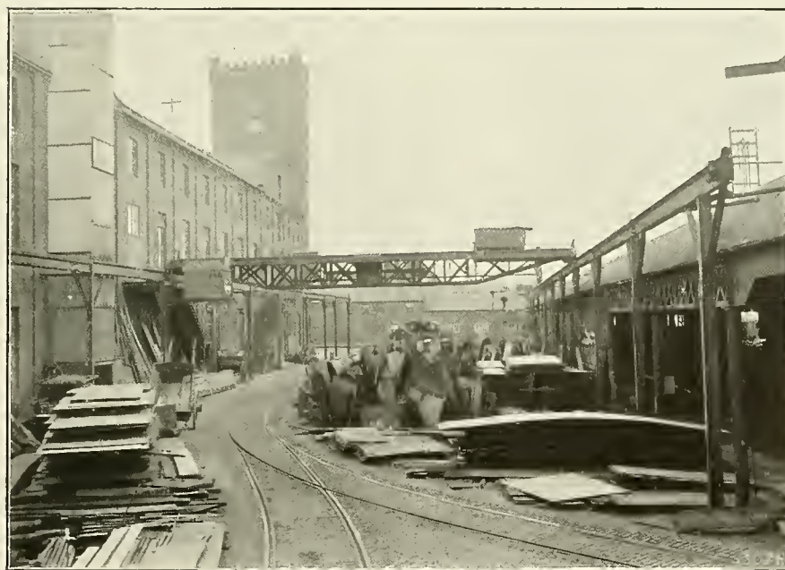
SHIPYARD PLATE RACKS, CARTSBURN YARD.
